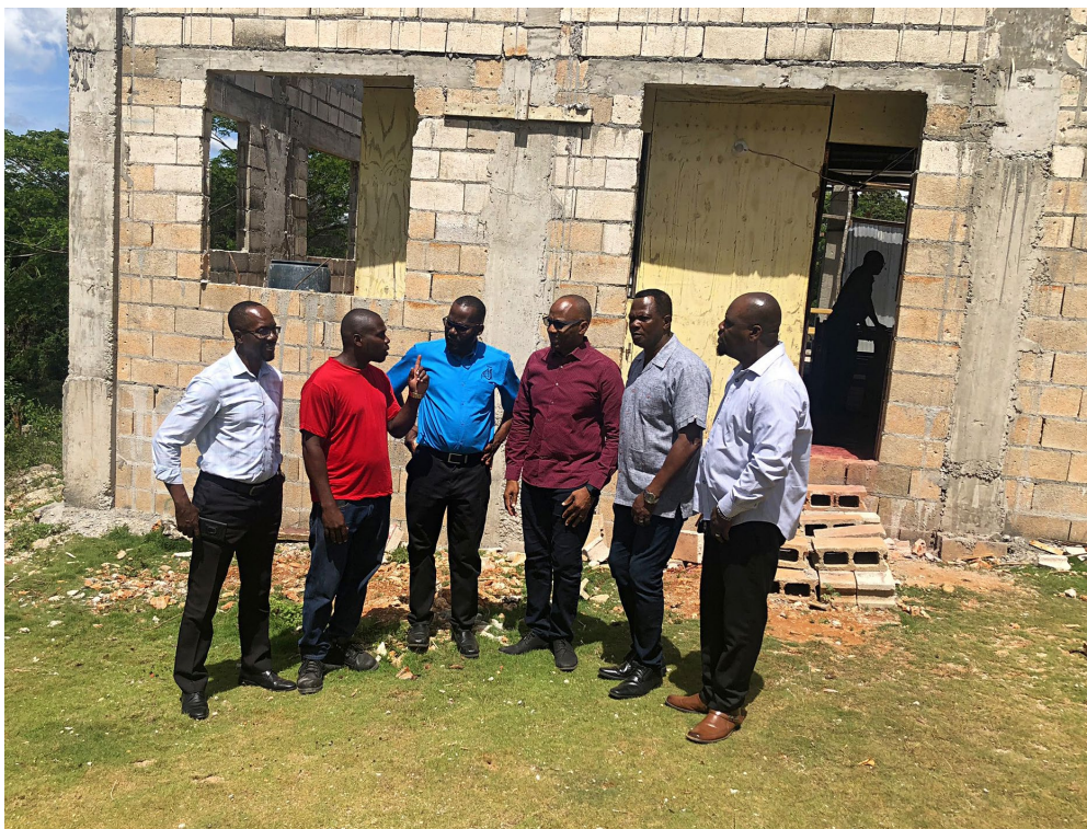
Lawrence Park under construction.
