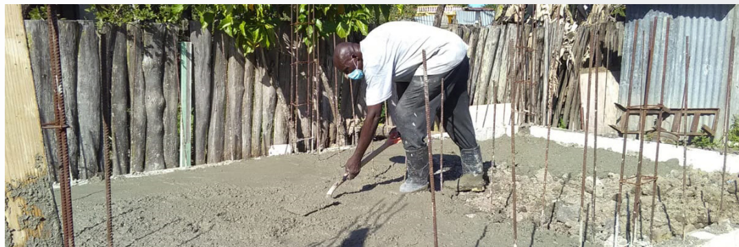
A construction project at the Annotto Bay Church.
